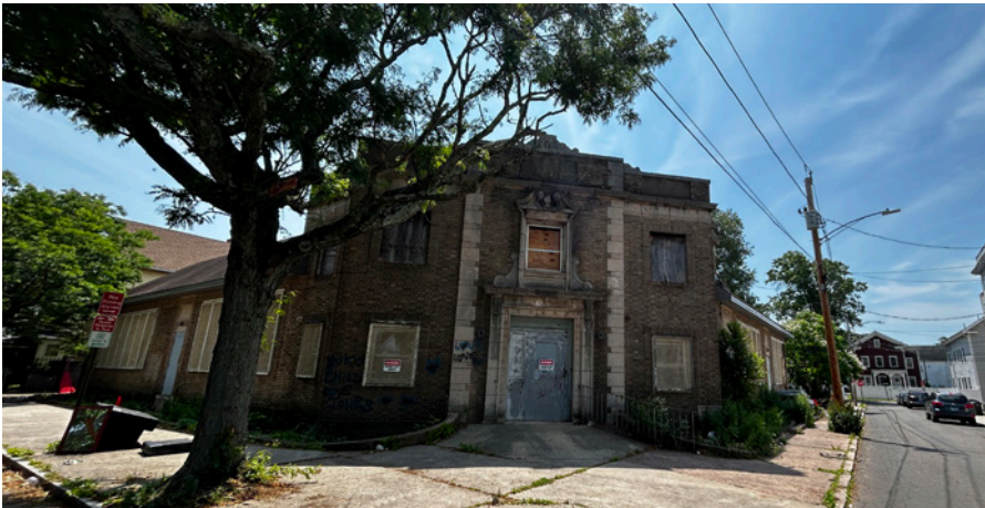
The renovation of the former Hill Cooperative Youth Center will provide much needed recreation space for Hill residents.
