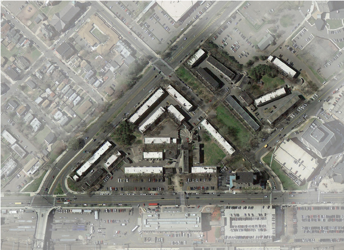
Church Street South Housing Project prior to demolition, 2014
