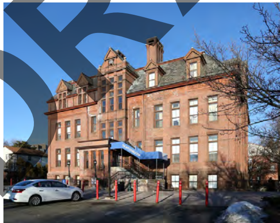
APT Foundation (Source: LoopNet)
