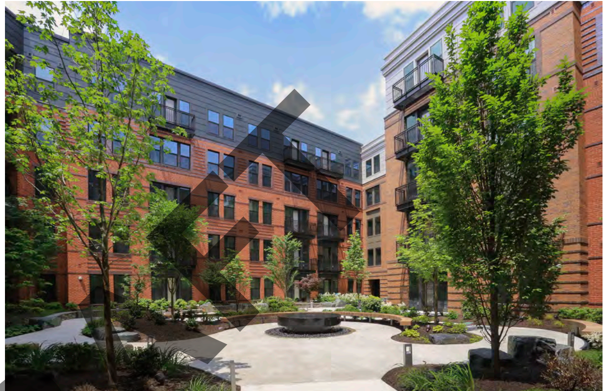
Figure 49: A landscaped residential courtyard
